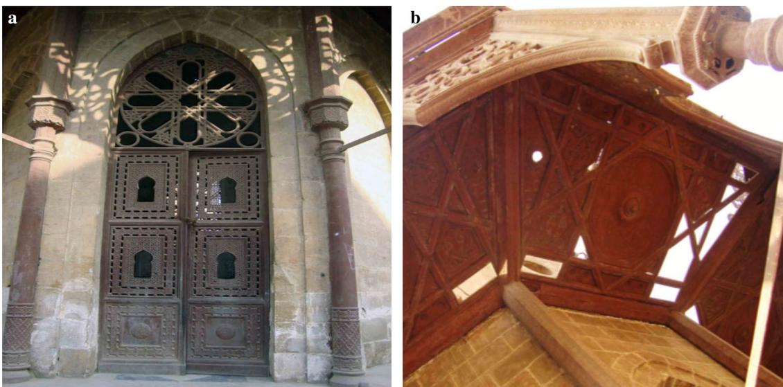
**Fig. 2** a Main gate of the tomb and b missing parts in the roof
