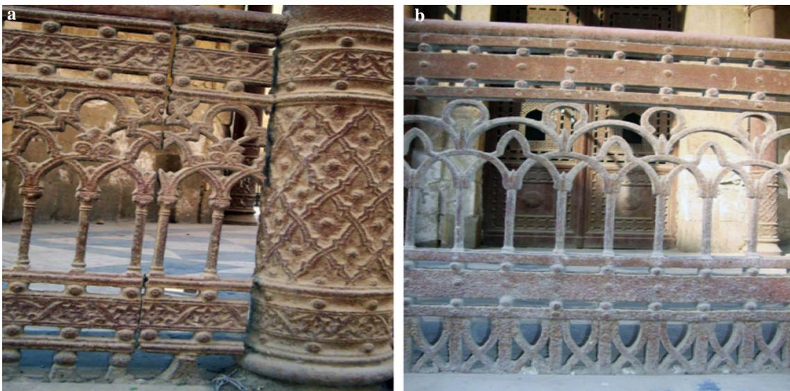
**Fig. 4** Dust particles covered the fine details of the decorative iron railings
