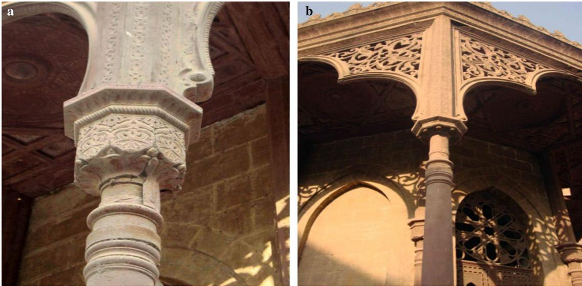
**Fig. 3** Missing parts in the decorative column
